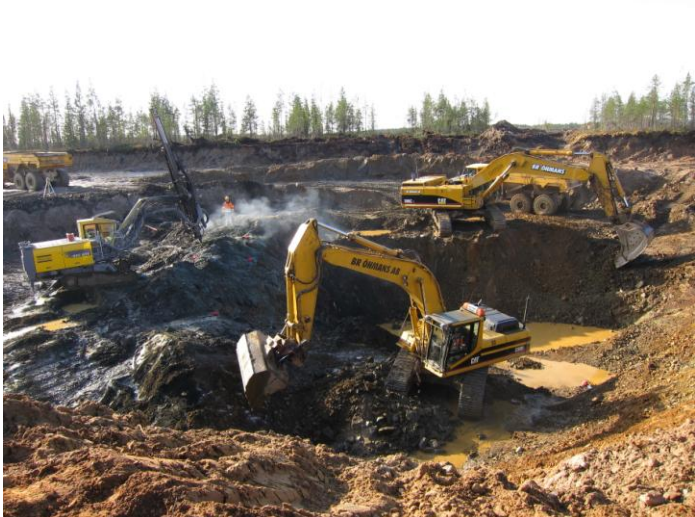
Overburden removal at Tapuli mine ore body. The work is ahead of schedule and is expected to be completed by September 2012.
