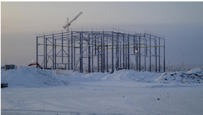
Erection of the steel work of the truck shop, January 2012
