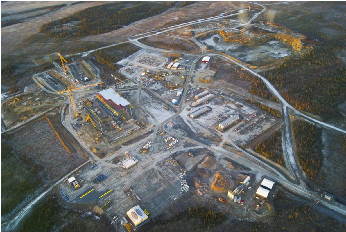
Figure 8: Construction at the Kaunisvaara Project site, November 2011
