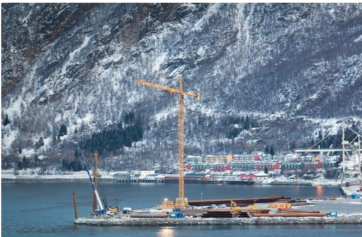
Figure 11: Construction work at the Fagernes Terminal in Narvik, Norway
